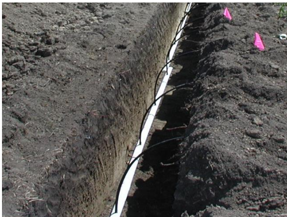
Figure 4: Buried water supply line connected to drip tapes
